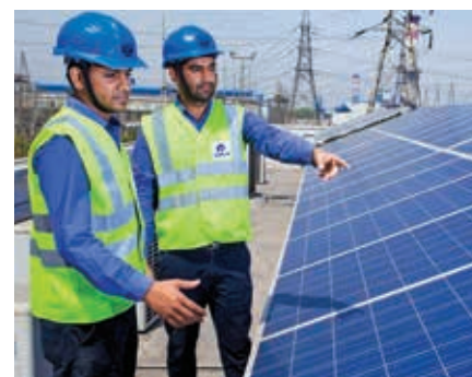
Solar panel installed in comprehensive building, BALCO
